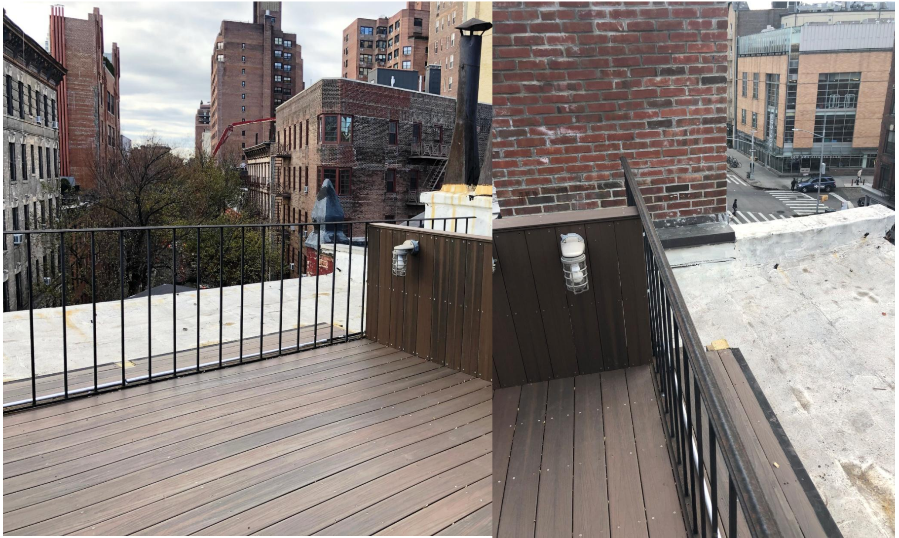
Bulkhead(s) On The Southern Side
