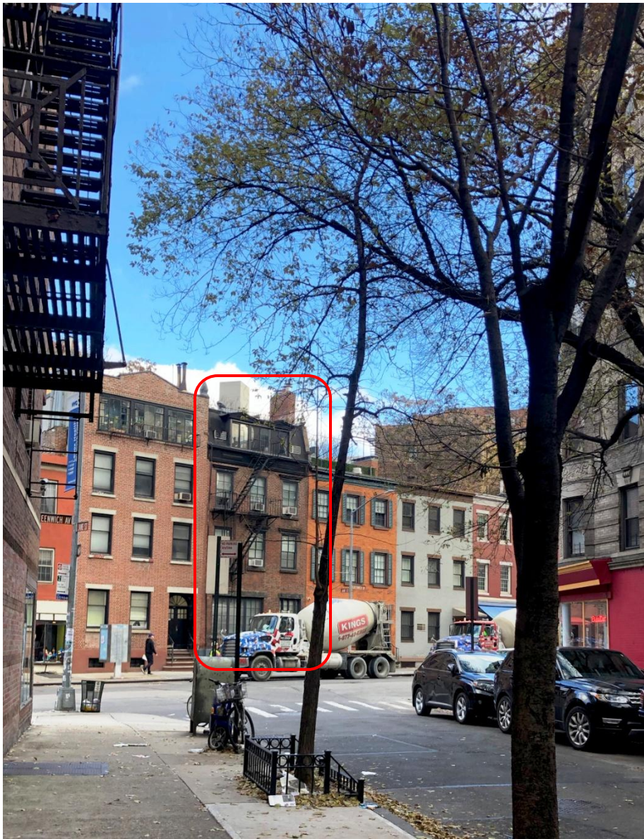
EXPOSURE OF BUILDING LOOKING FROM JANE ST. BOUND ON GREENWICH AVENUE
