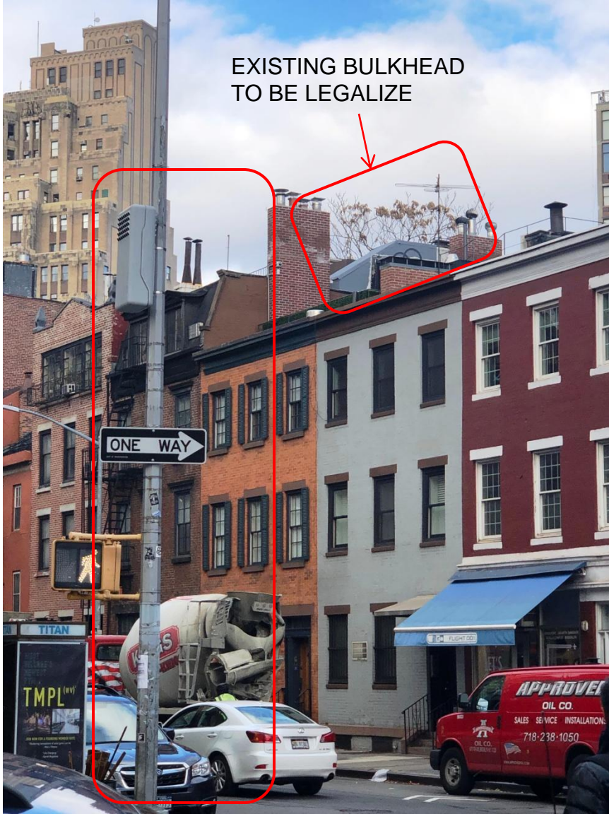
EXPOSURE OF BUILDING LOOKING NORTH BOUND ON GREENWICH AVENUE
